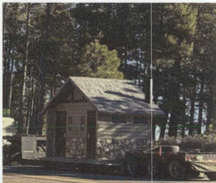
This beautiful new public restroom was made possible by the FLAP grant. What a great addition for mountain visitors!
