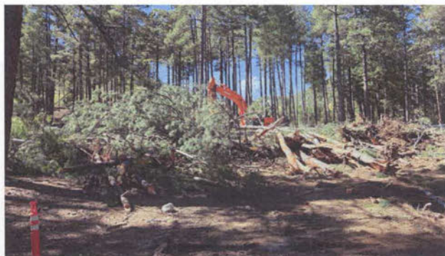
Tree clearing near the old schoolhouse
