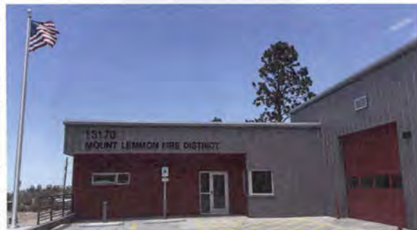
The new MLFD station
