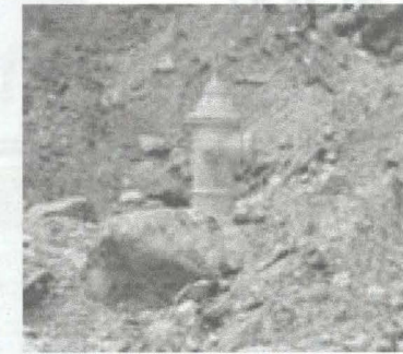
Left: one of three new fire hydrants installed along Tucson Avenue as part of the pipeline replacement project. Right: newly installed water meters. (Photos by Doug Mance.)
