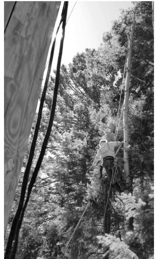
Asplundh employee climbs a tall aspen to remove encroaching limbs that could threaten Trico's transmission line to Mt. Lemmon. | Photo courtesy Trico Electrical Cooperative
