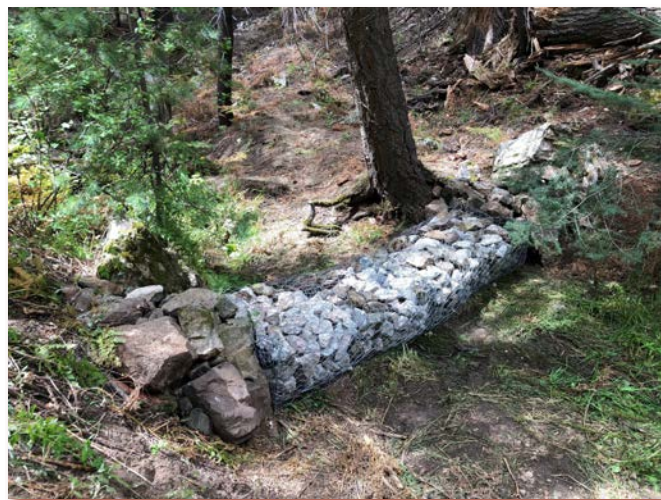
New check dams were installed in Upper Sabino Creek.
