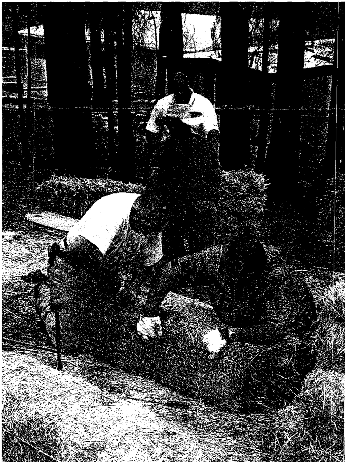
NeighborWise Section Leaders Alex Carrillo and Bill Piatkiewicz wrap straw bale with chicken wire as an NRCS worker helps Tom Alfonso begin another bale. These straw bales were used to construct erosion check dams in the demo project just south of Zimmerman Elementary School.
